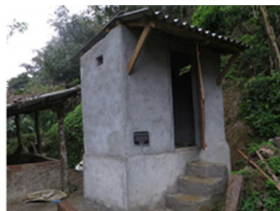
Toilet built with support from LIXIL
