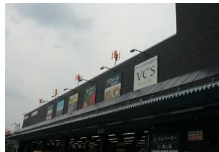
▲ Solar panels and wind turbines at Super Viva Home
