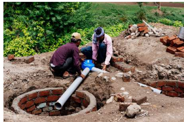
Installing SATO V-Trap toilet
