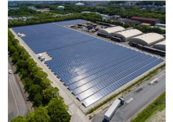
LIXIL Chita SOLAR POWER generated approx. 6,700MWh in FY2016
